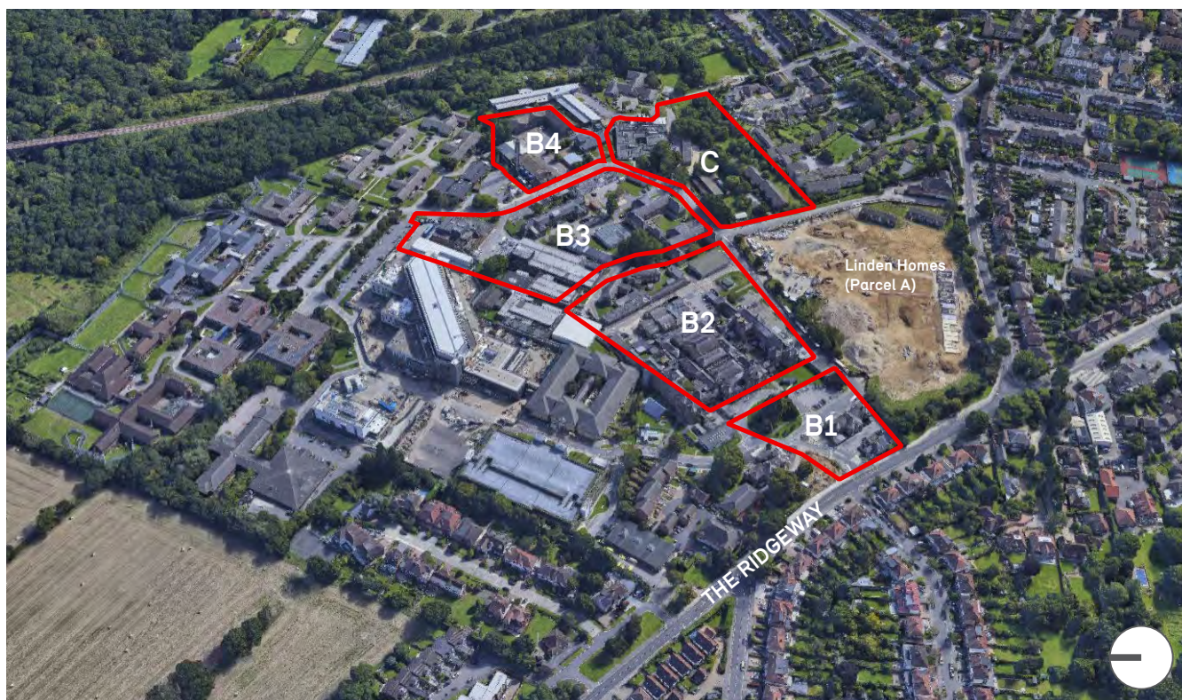
FIG 2 - AERIAL PHOTOGRAPHS FROM SOUTH AND WEST
