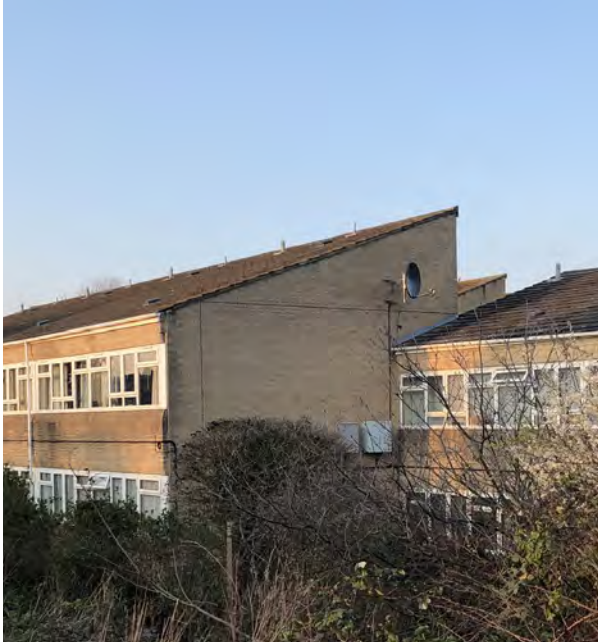
ROOF FORMS ADJACENT TO SITE
