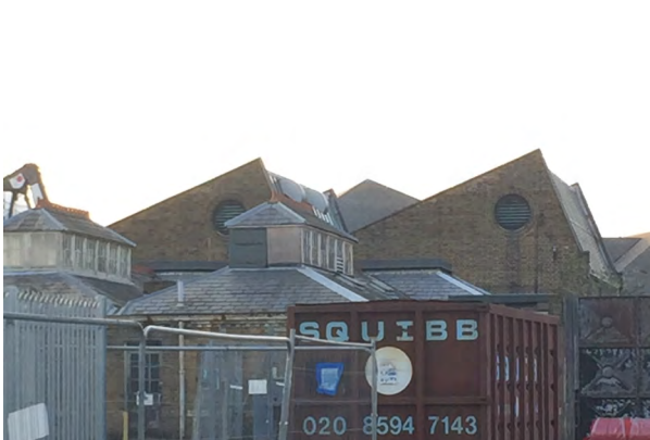
HISTORIC ROOF FORMS ON SITE
