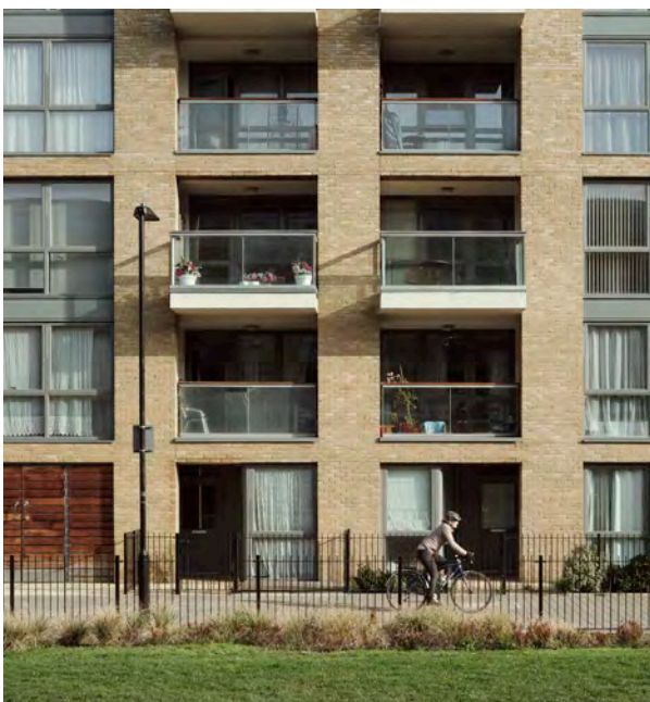
SEMI-RECESSED BALCONY PACKINGTON ESTATE - PTE
